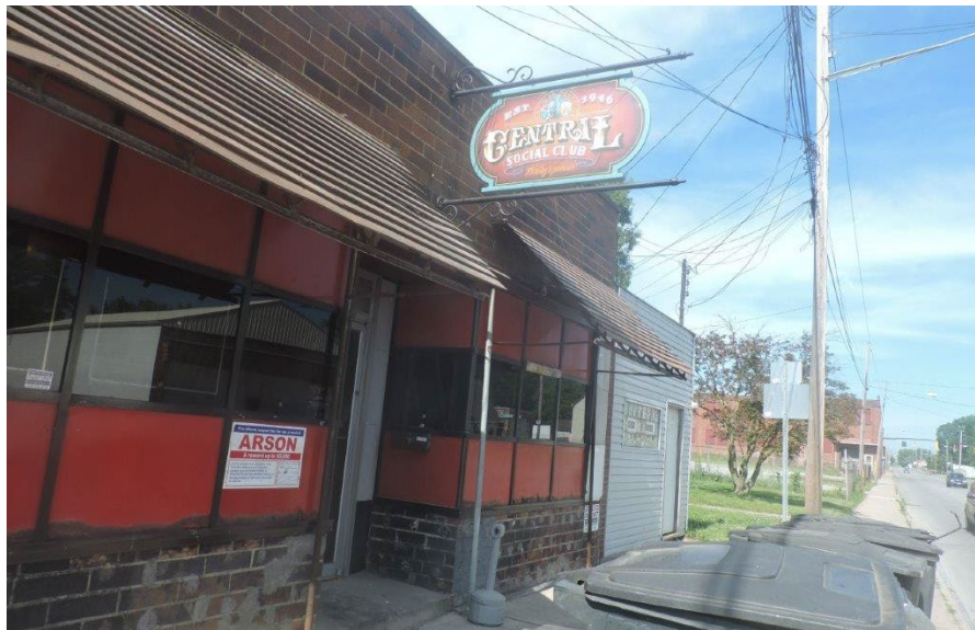
The scene of a fire at 1171 W. Market St. in Warren (Trumbull County).
