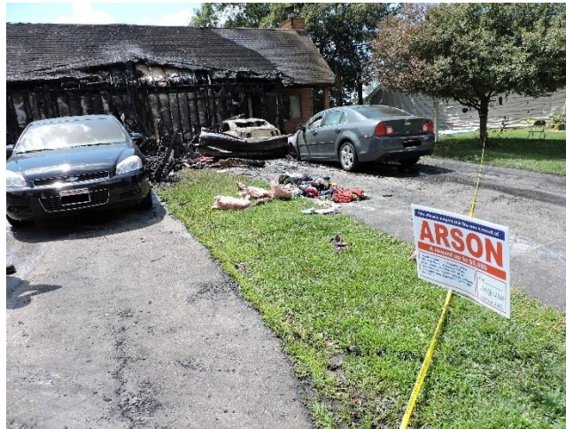
Fire damage to duplex on Copperfield Drive in Chillicothe.
